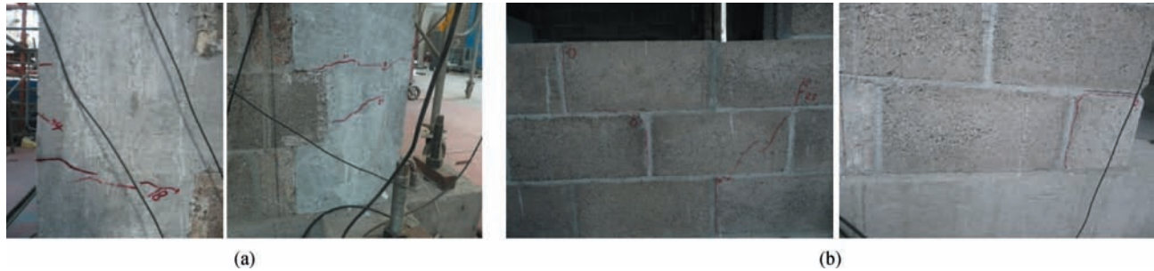
Fig. 14 Failure pattern of precast RAC block masonry structure. (a) Tie column; (b) masonry wall
