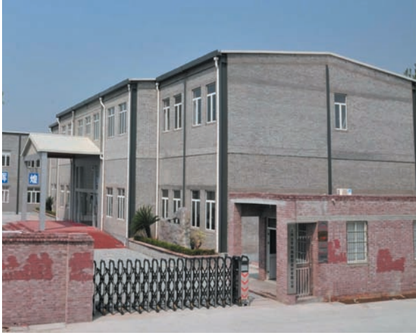
Fig. 20 Office building using recycled aggregate bricks
