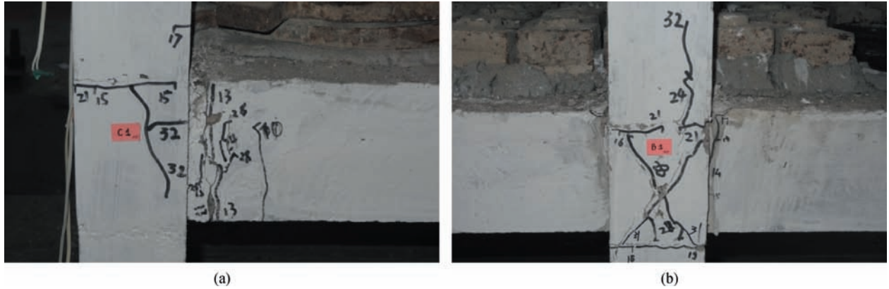
Fig. 8 Failure pattern of the precast RAC frame structure. (a) Beam; (b) column and joint
