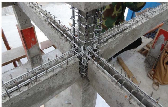
(e) Typical configuration of the assembled joint
