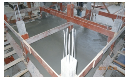
(c) Pouring RAC for joints and slabs
