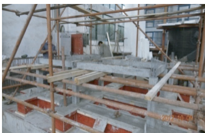
(a) Lay up precast RAC beams and columns
