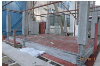
(b) Welding rebar of joints
